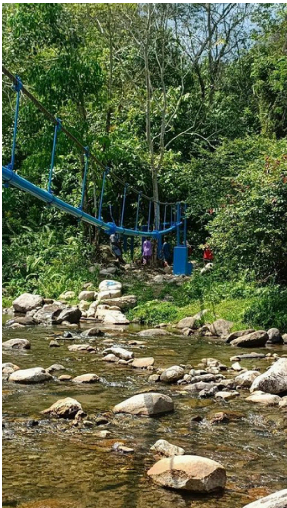
Figure 26 · Drinking Water Supply System (SPAM) piped network
