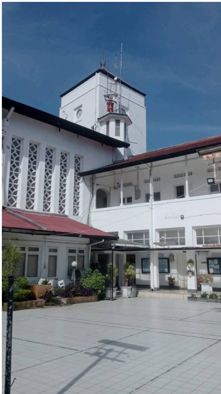
Figure 35. Early warning sirens in Padang City
