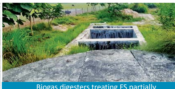
Biogas digesters treating FS partially along with cowdung
