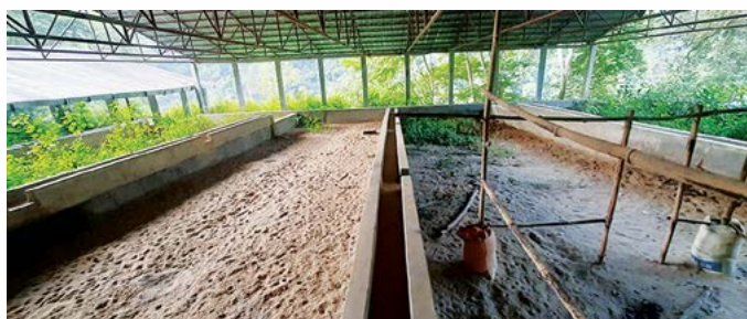
Partially completed FSTP of Vyas
