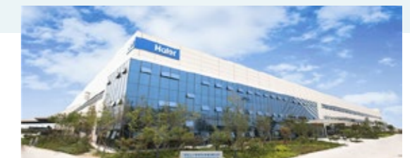
Haier's washing machine factory in the Qingdao Area of the China (Shandong) Pilot Free Trade Zone. [Photo/WeChat account: qdgx2019]
